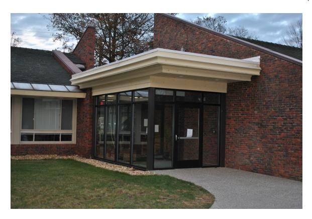
This facility is a Single-story, 628sf +/-, structural steel frame and aluminum storefront glass building, approximately 15-feet high. This connector building was designed to reduce the schools energy consumption, as well as provide a gather and study area for the students. While providing a well light, warm and inviting appearance that would not overwhelm the original two classroom buildings.
